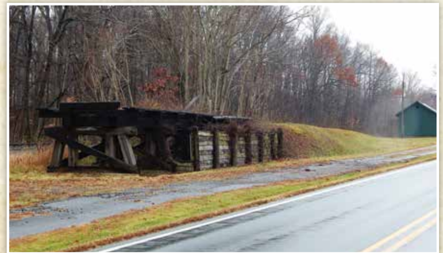
Fig. 6. The Montpelier hopper car trestle, all that is left of the small rail yard that once existed here. The Detrick & Bradley fertilizer warehouse is in the right background. The NS main line runs along the edge of the trees. Photo courtesy of Bernice Walker.
