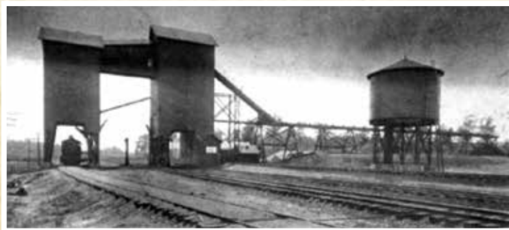
Fig. 4. The original frame Weyburn coaling tower that went into operation in 1905. In the 1930s, it was replaced by an even bigger concrete tower. In 1953, with railroads switching to diesel-electric locomotives, that tower was removed with explosives. Photo courtesy of Duff Green and the Orange County Review .
